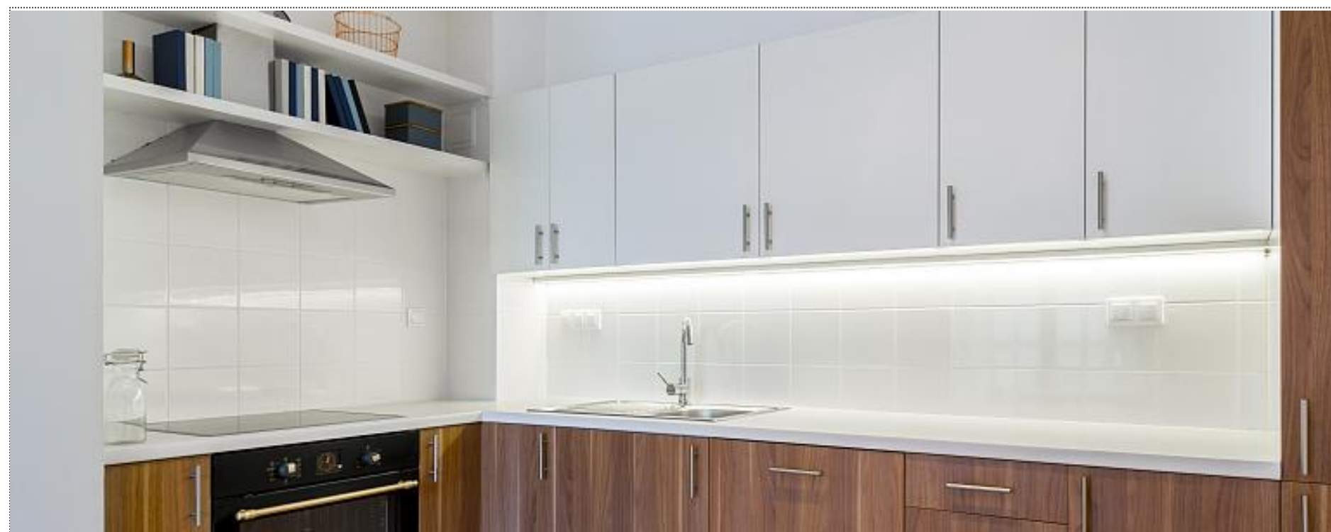
Kitchen lighting 厨房照明
